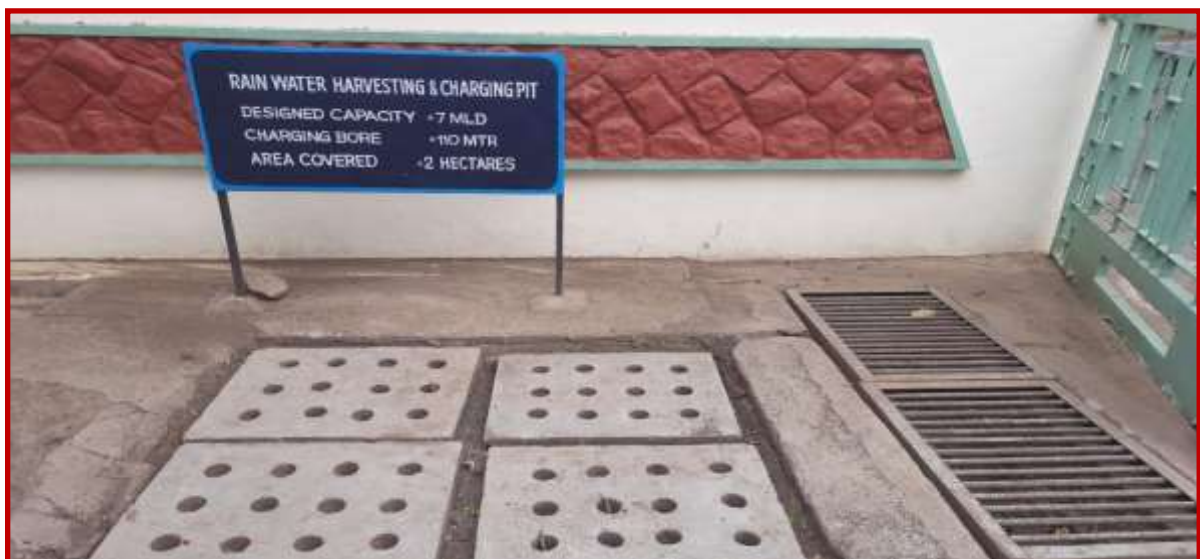
Fig.3: Sample Rain Water Harvesting (RWH): Storage and Name Board Representation
